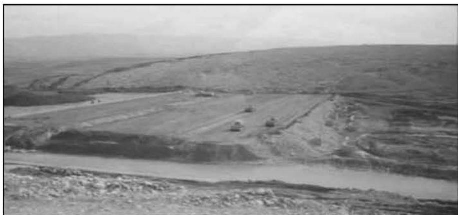
Figure (37) Spill way in kurdistan region
